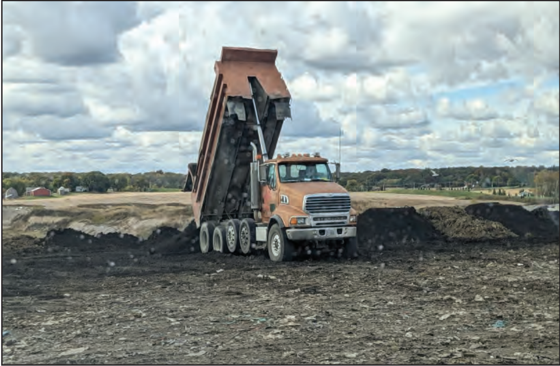
Tipping landfill direct soils with too much bulk waste for cover
