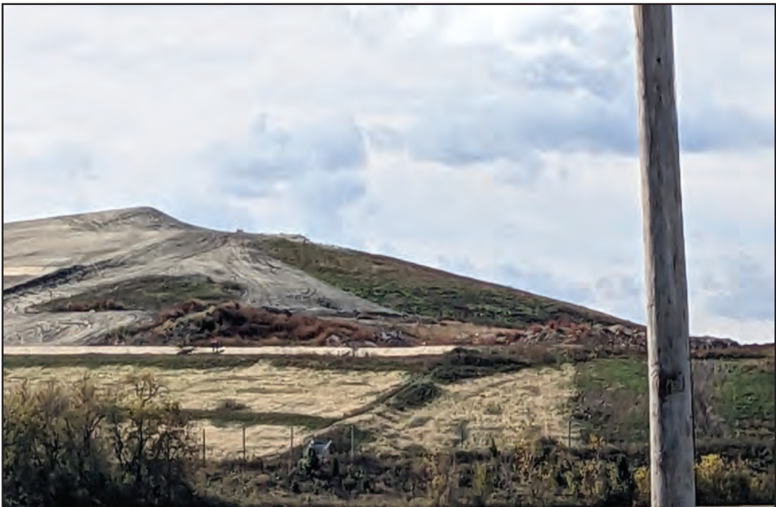
Armoring on new cap project
