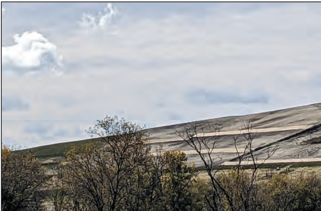
Armoring on new cap project
