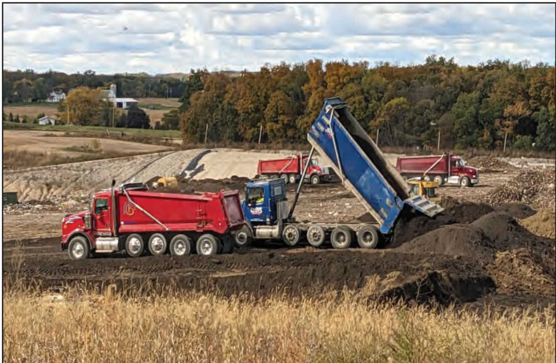
Tipping landfill direct soils with too much bulk waste for cover
