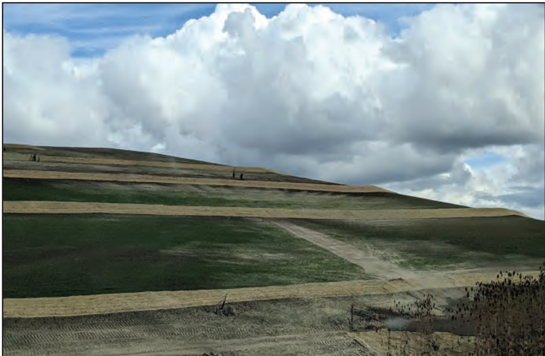
Armoring extended to previous cap project
