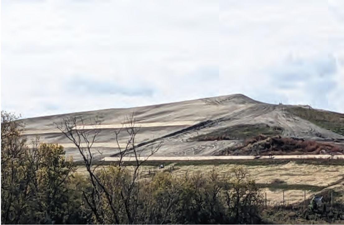
Cap conditions viewed from the East
