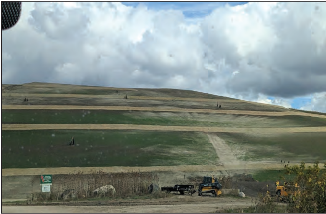
Armoring extended to previous cap project
